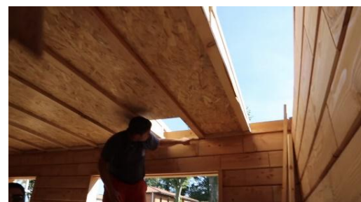
Gambar 7. Roof framing & setting
