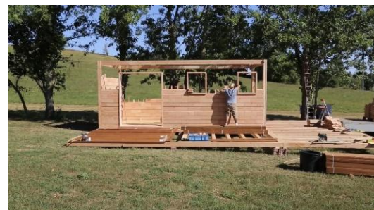
Gambar 5. Wall setting & sheathing
